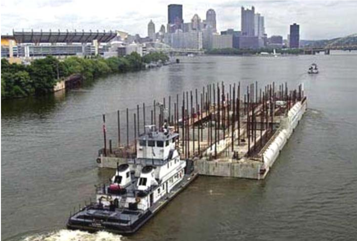
a. Open-river transport of a dam segment
