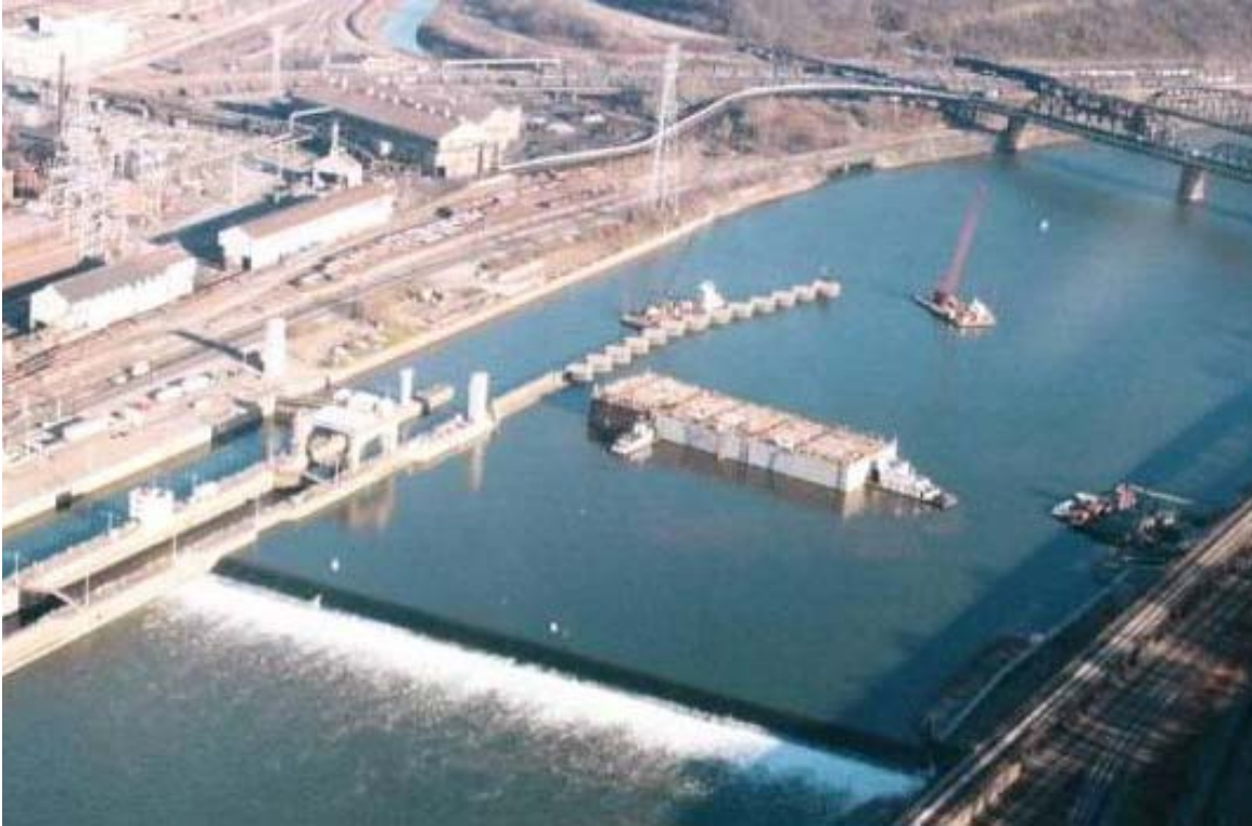
a. Initial positioning of dam Segment 1
