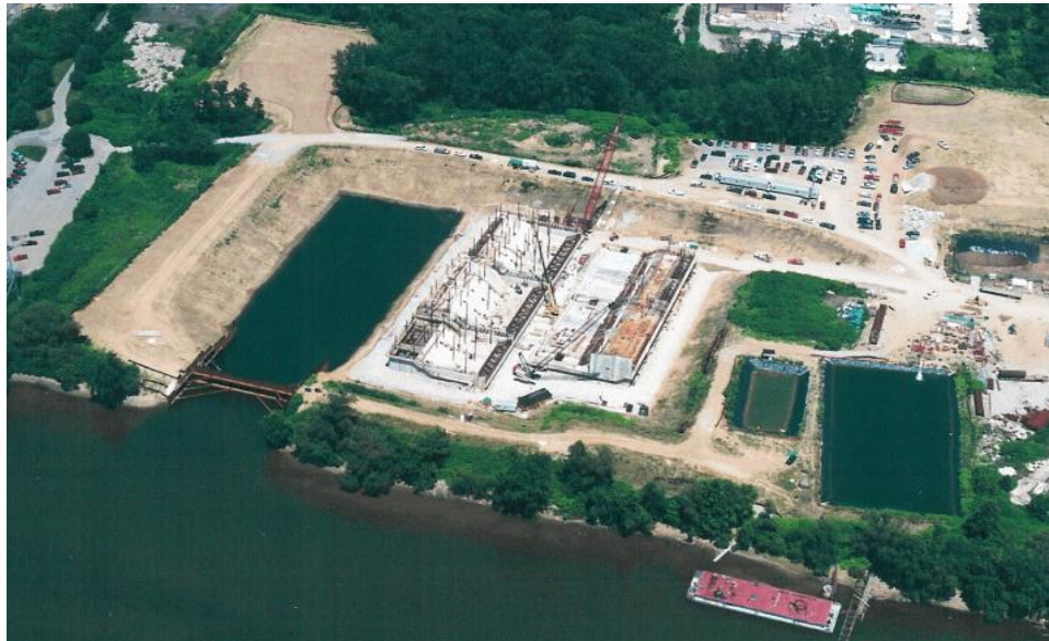
a. Prefabrication site, Leetsdale, PA
