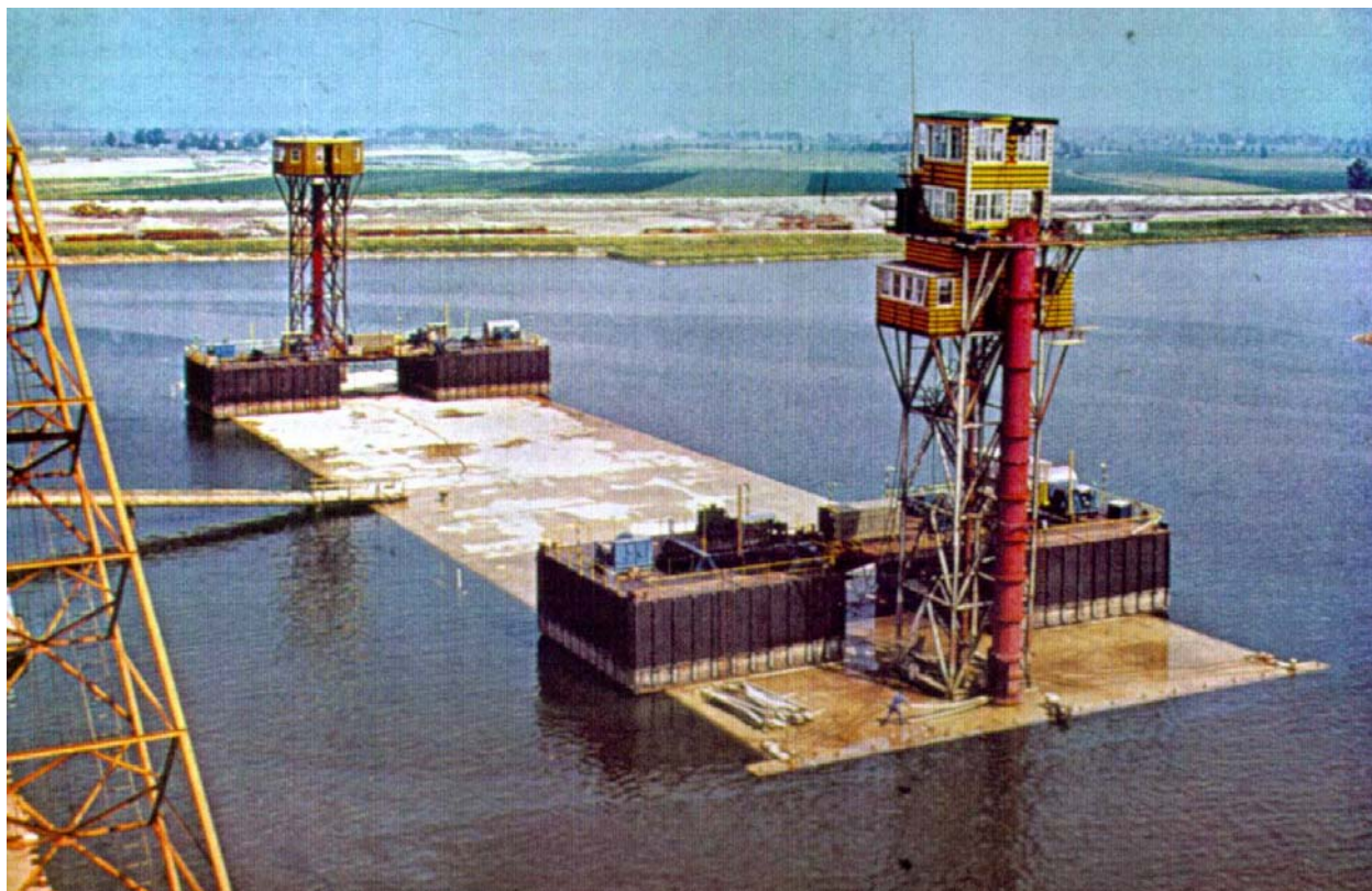
Figure C-8. Typical European-style concrete immersed tube segment
