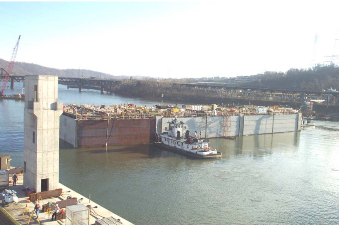
b. Close-up of initial positioning of dam Segment 1 Figure C-13. Positioning of the first segment for Braddock Dam
