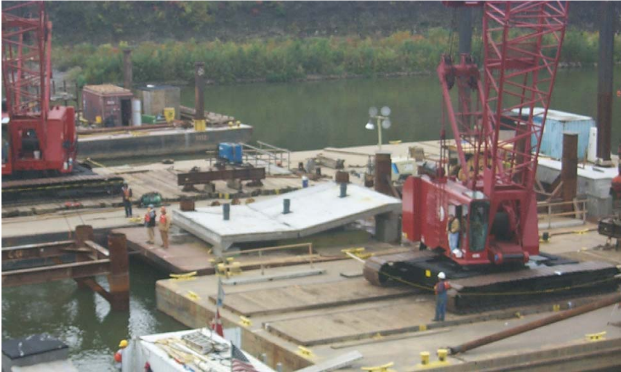
Figure C-14. In-the-wet tailrace panel installation for Braddock Dam
