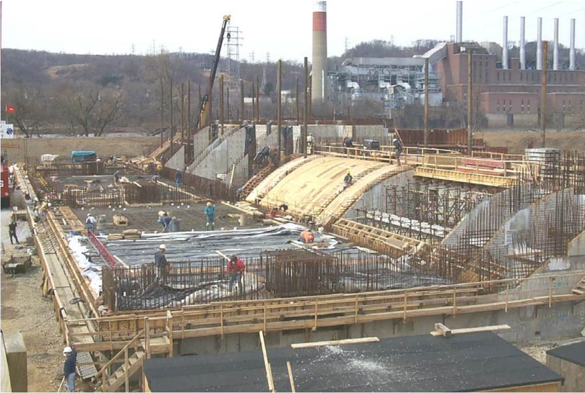
a. Construction of dam Segment 1 within the two-level casting basin
