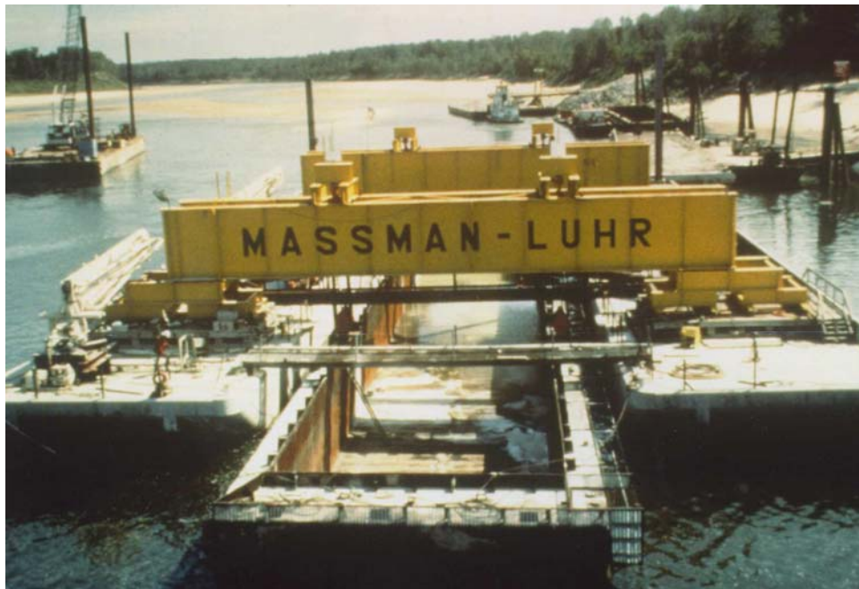
Figure C-6. Emergency repair operations for the Wilbur Mills Dam
