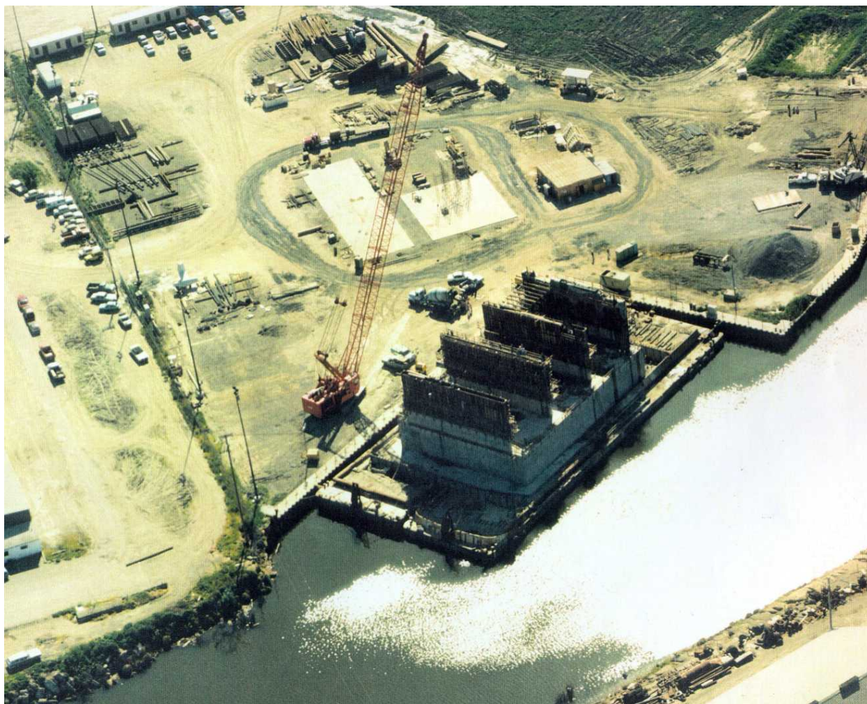
Figure C-1. Radial gate structure under construction for the Montezuma Slough Salinity Barrier
